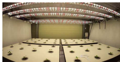
Plant-centric Spectrum LED (LM301H EVO) Full White (437nm) + Red (660nm)
